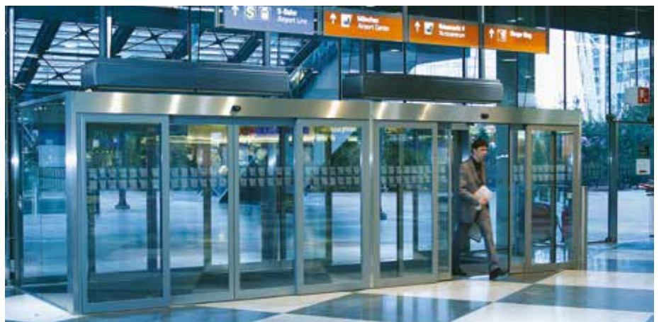
Smoke-protection doors, entrance area, MUC
