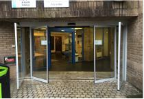
Geographical and Earth Sciences Department in Glasgow University. This is the record TOS - Total Breakout system which is a sliding door with break out capacity suitable where emergency passage may be required.
